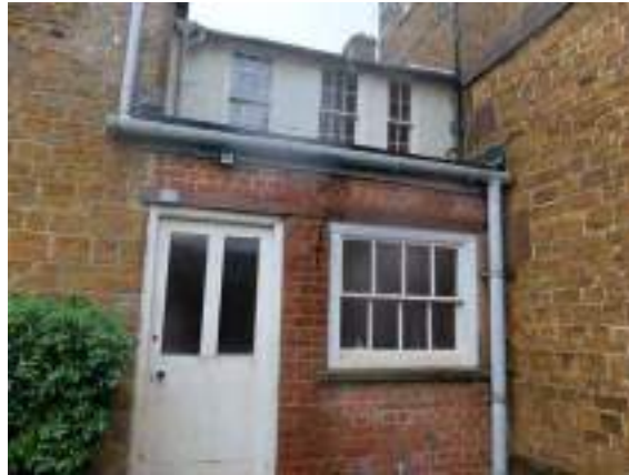
Fig.22 Infill brick section rear service modern fenestration
