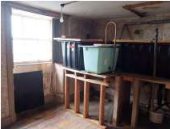
Fig.65 S3A shutters and 'garret' windows intact.
