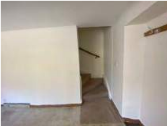
Fig.50 Winder stairs to first floor G5
