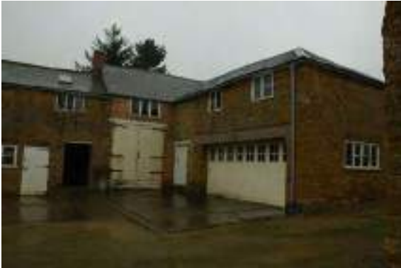
Fig.25 Garage east side of yard
