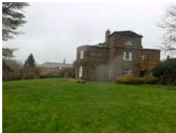
Fig.28 South west elevation with additional attic storey
