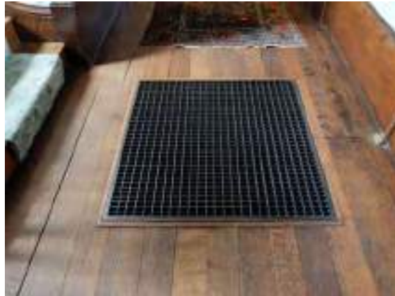
Fig.34 Ventilation grill installed 1930s
