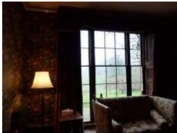
Fig.36 G10 Full height tripartite sash windows overlooking garden
