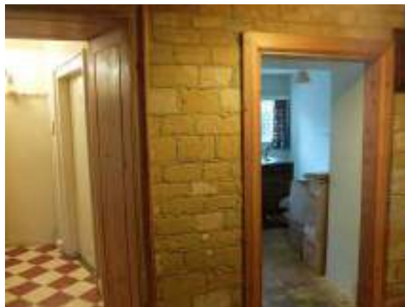
Fig.53 Service corridor exposed stone blockwork
