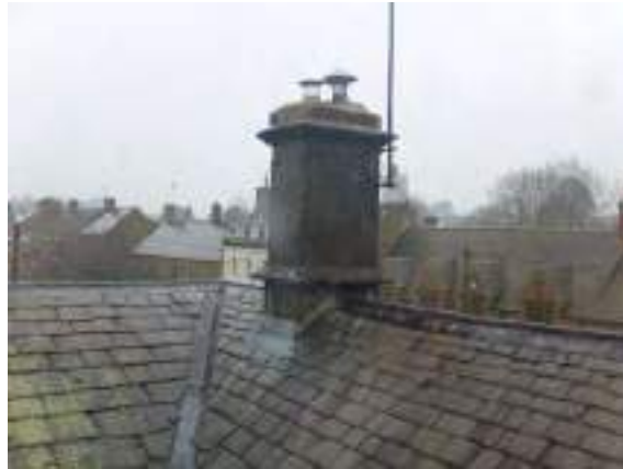
Fig.32 Smoke blackened ashlar chimney stack over service range
