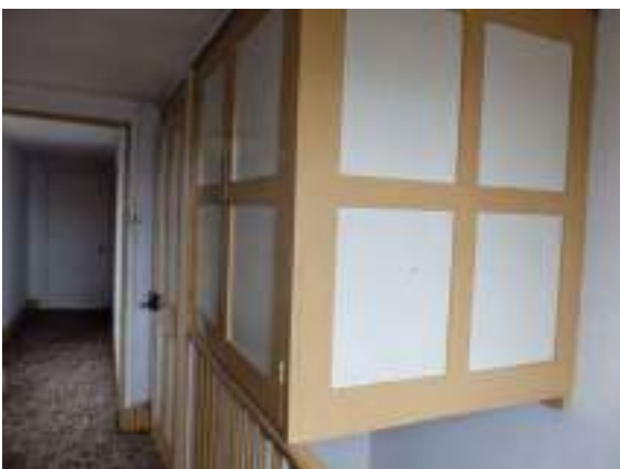
Fig.63 Attic corridor with cupboard over stairwell
