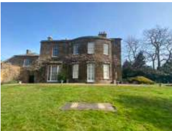
Fig.27 Rear west facing principal elevation
