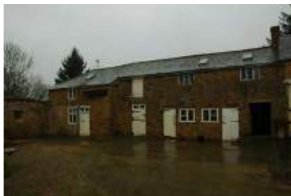
Fig.20 Former stable and hayloft north side of yard
