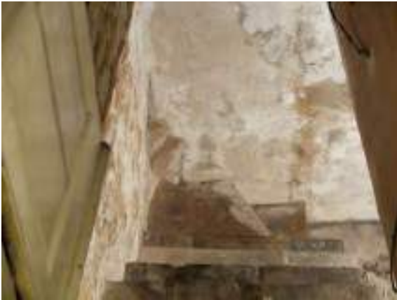
Fig.41 C5 cellar steps evidence of earlier steps in left corner
