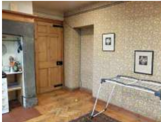
Fig.47 Blocked doorway to cellar? Kitchen G8
