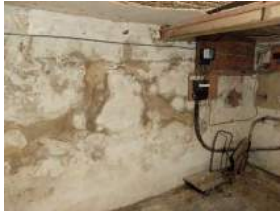
Fig.42 C5 plastered walls, concrete slab floor and RSJ
