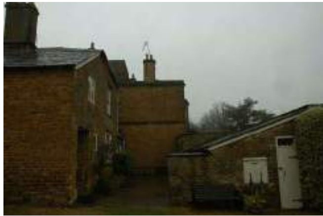
Fig.24 Service range and outbuildings
