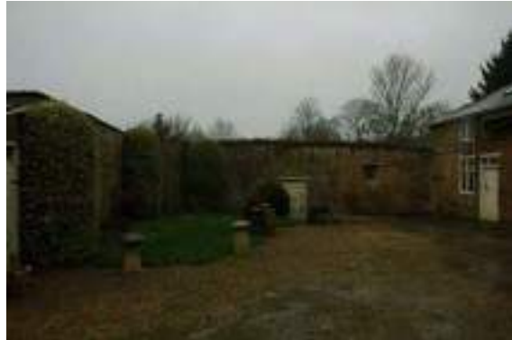
Fig.26 Walled kitchen garden entrance contiguous with outbuildings
