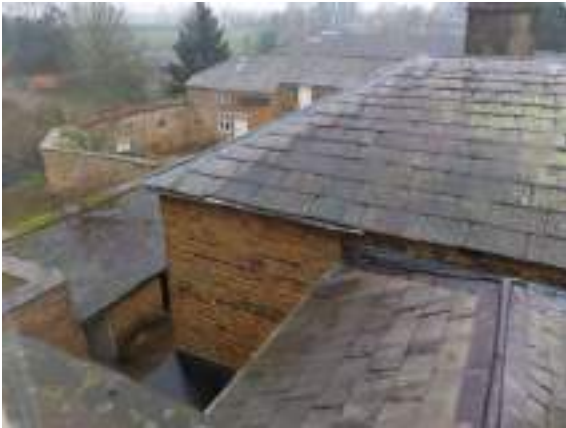
Fig.31 Slate roofs over service range
