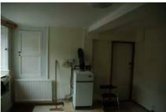
Fig.48 Chimney recess cupboard G5
