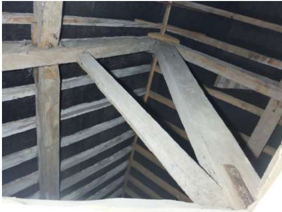
Fig.116 - 117 Butt-purlin roof construction with machined timber king post roof truss and metal plate reinforcement
