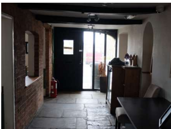
Fig.55 - 56 G2 Carriage entrance, flagged floor and 'cobbled area' to one side. Door and glazed screen to front and half-glazed doors and window to rear yard. Reinforced cross beams, and exposed brickwork with a mix of contrived and re-purposed openings lining the passage.
