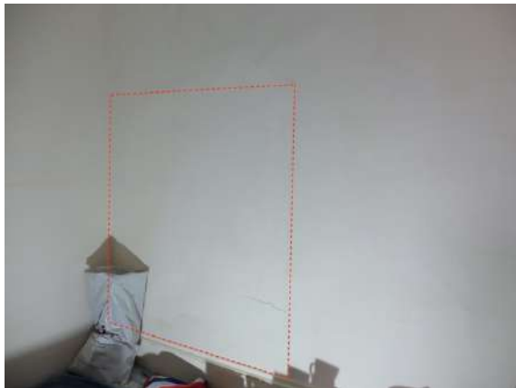
Fig.81 F3 rear wall with former opening indicated
