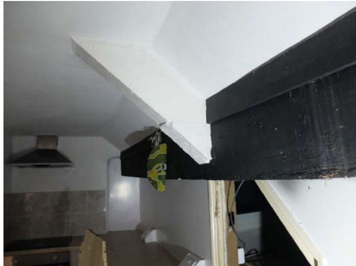
Fig.113 S5 Exposed truss feet and purlin
