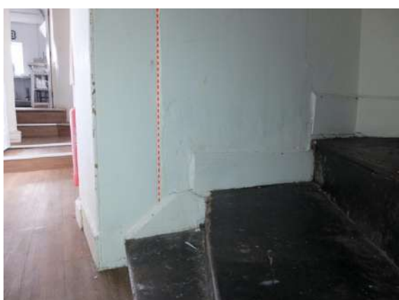
Fig. 85 - 86 F4 Wall extended at base of stairs and recess to side wall
