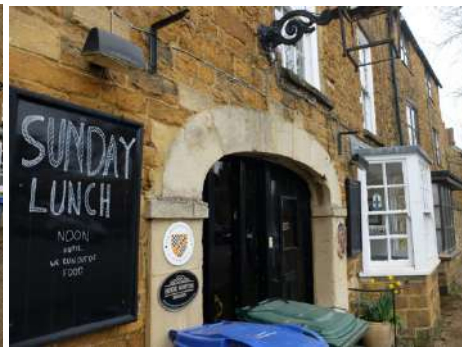
Fig.30 Depressed arch in ashlar stone
