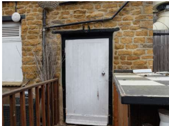
Fig.69 - 70 Side elevation - rendered to sill height, concrete lintel to half-glazed door and timber lintel to plank door. A horseshoe affixed to the lintel may indicate former use as a stable.
