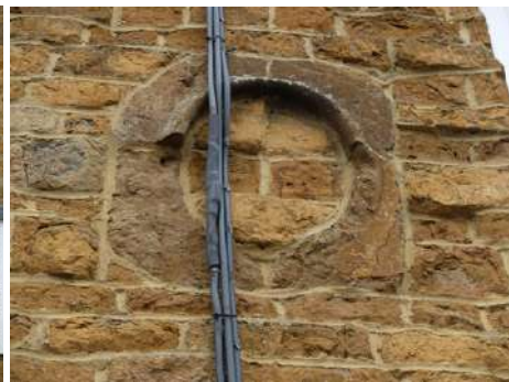
Figs.31 - 33 Decorative oval plaques harmed by badly positioned cabling- later infill particularly noticeable on the lower of the two.
