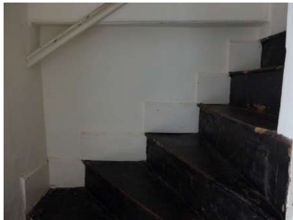
Fig.83 - 84 F4 C19 Stained timber treads to second floor - boxed-in C20 baluster and newel post
