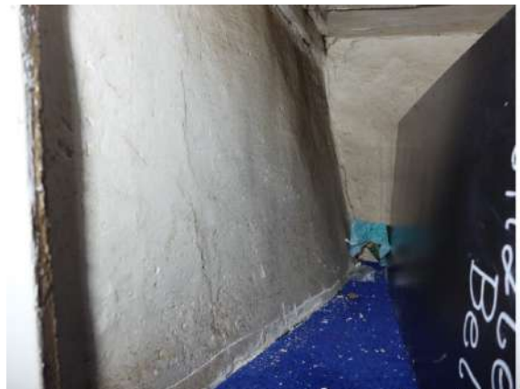
Fig.91 - 92 F5 cupboard interior - uneven masonry, curvature to the chimney breast side wall denotes C17/C18 staircase
