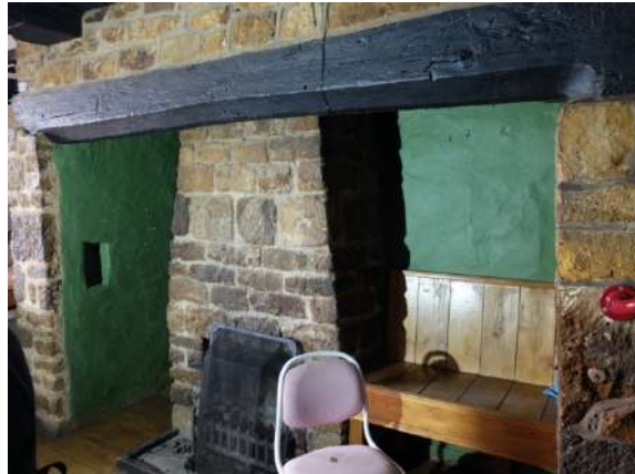
Fig.52 'Iglenook' with inserted chimney breast and fire grate
