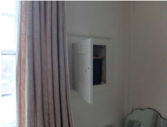
Fig.75 -76 F1 Wall cupboard with safe inserted and outline of oval panel on the back wall.
