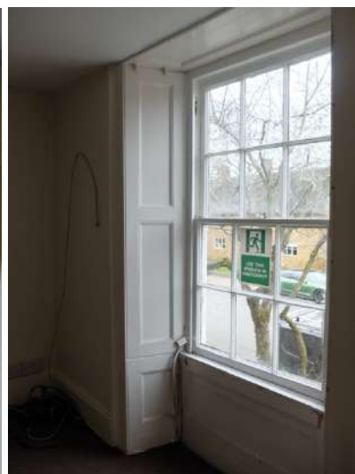
Fig.80 F2 Panelled shutter boxes
