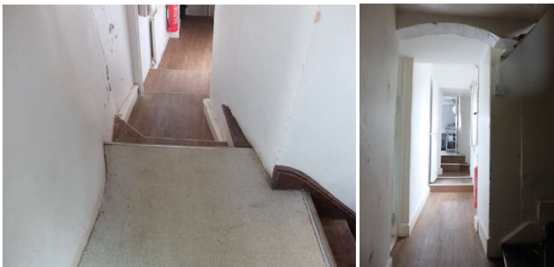
Fig.95-96 F8 Three changes in level landing area - seen from east to west and then in reverse - note bottom step to concealed staircase RHS of Fig.93
