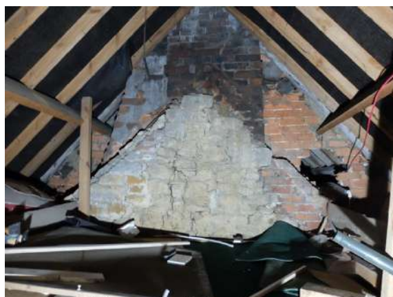
Fig.115 Fabric in roof void demonstrating lower roof pitch
