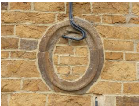
Figs.31 - 33 Decorative oval plaques harmed by badly positioned cabling- later infill particularly noticeable on the lower of the two.
