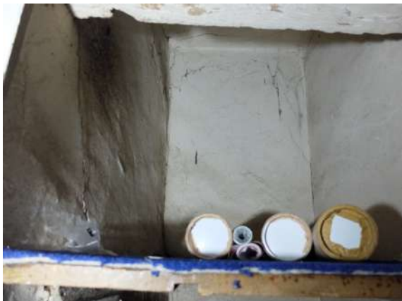
Fig.91 - 92 F5 cupboard interior - uneven masonry, curvature to the chimney breast side wall denotes C17/C18 staircase
