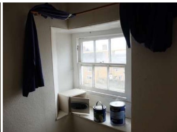
Fig.104 - 105 S1 Sash windows inset with deep reveals - side wall angled to accommodate walk-in cupboard from S4
