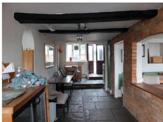
Fig.55 - 56 G2 Carriage entrance, flagged floor and 'cobbled area' to one side. Door and glazed screen to front and half-glazed doors and window to rear yard. Reinforced cross beams, and exposed brickwork with a mix of contrived and re-purposed openings lining the passage.
