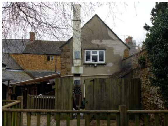
Fig.38 Infill brickwork and disturbed stonework and lintel Fig.39 End gable rendered with large extraction flue
