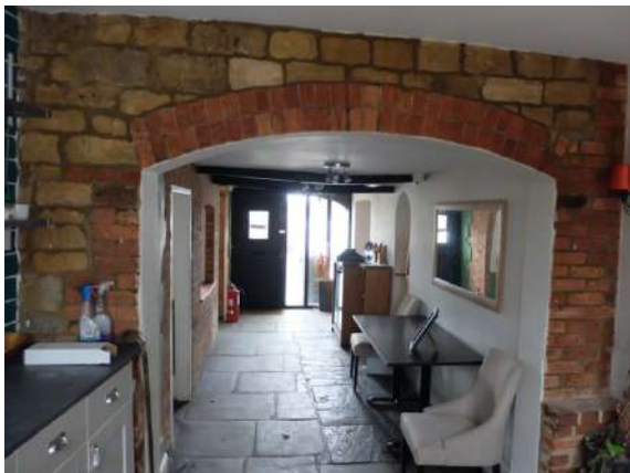
Fig.63 - 64 G5 Brick and stone 'external' wall of the main range. Lobby entrance to WCs and rear southern range (stables)
