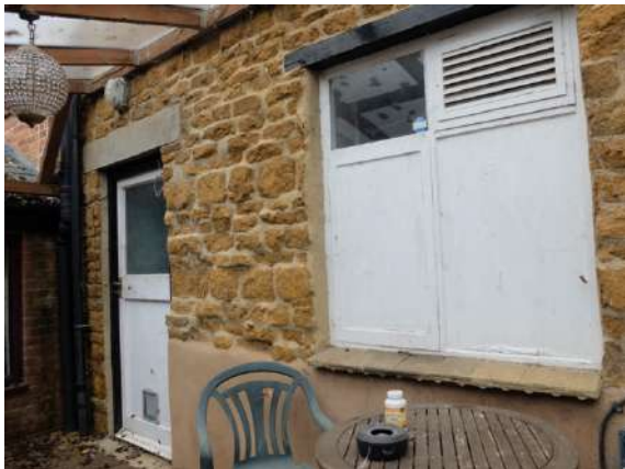
Fig.69 - 70 Side elevation - rendered to sill height, concrete lintel to half-glazed door and timber lintel to plank door. A horseshoe affixed to the lintel may indicate former use as a stable.
