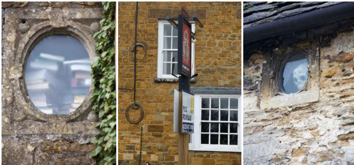
Fig.120 - 122 Early C18 Oeil-de-boeuf windows compared to those found on the front elevation of the Crown and Tuns.
