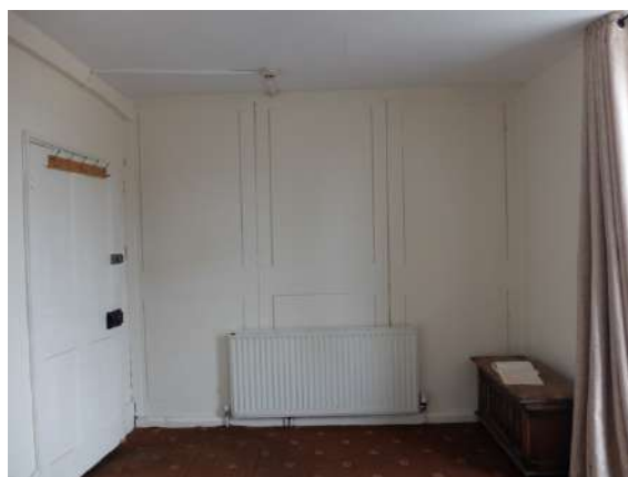
Fig.74 F1 Panelled partition wall dividing the front rooms
