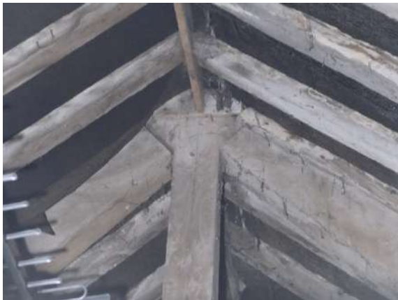
Fig.118 Ridge plate or plank set square
