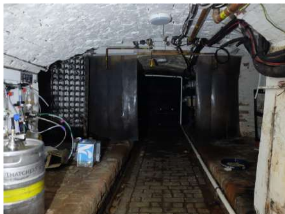
Fig.48 Brick-lined cellar with drainage channels and plinths
