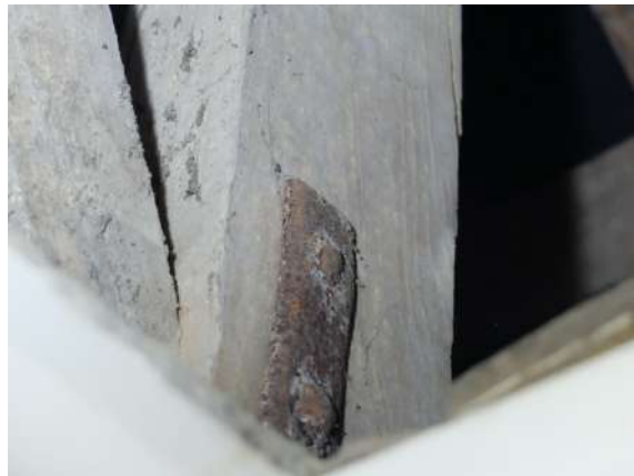
Fig.119 Iron plates and bolts used alongside pegs.
