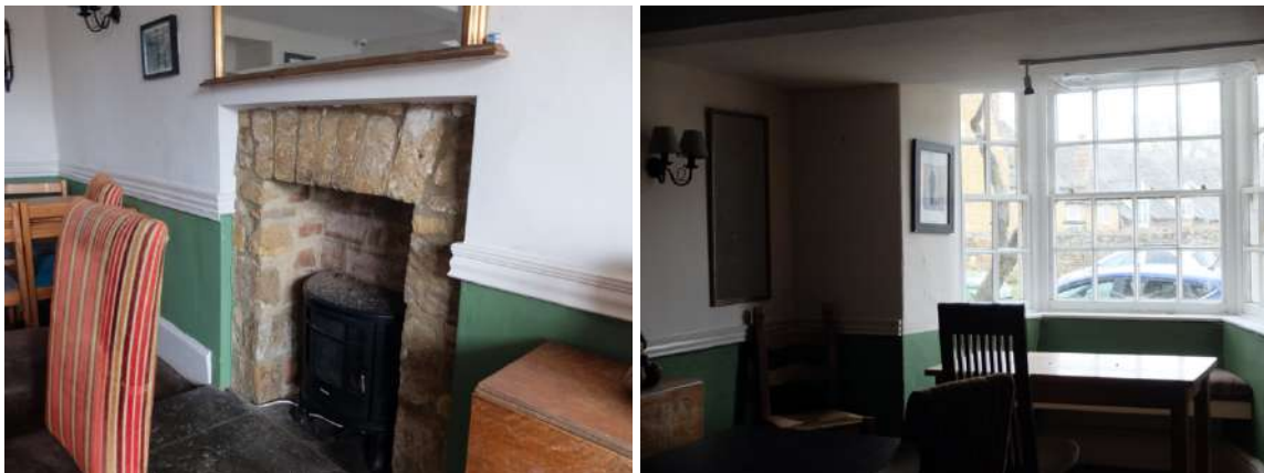
Figs.59 - 60 G3 Stone fire surround and returns, with stone soldier course lintel, brick infill at rear and modern wood burner. Boxed in cross beams, possible steels and matching bay at the front.
