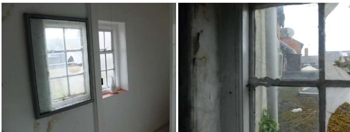
Fig.93-94 F6 Casement divided by partition - metal casement LHS and modern timber RHS - turnbuckle catch c.1700
