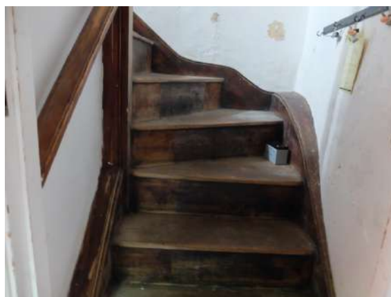
Fig.72 F9 Stained timber stairs plain nosed treads
