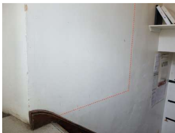
Fig.98 F9 Top of stairs uneven wall section indicated
