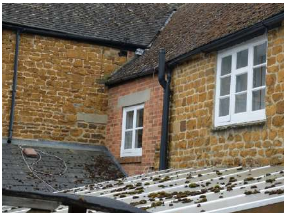
Fig.38 Infill brickwork and disturbed stonework and lintel Fig.39 End gable rendered with large extraction flue
