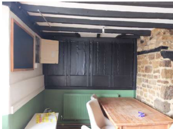
Fig.54 Note trimmed ceiling joists, small cupboard to front
