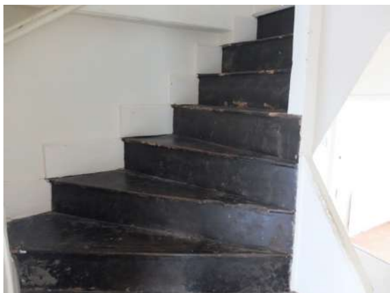
Fig.83 - 84 F4 C19 Stained timber treads to second floor - boxed-in C20 baluster and newel post
