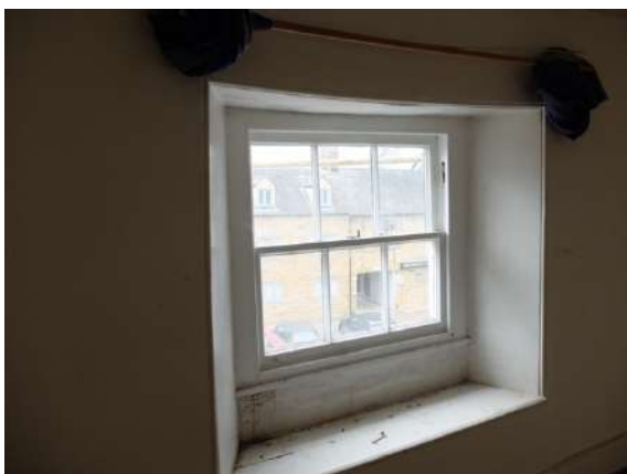
Fig.104 - 105 S1 Sash windows inset with deep reveals - side wall angled to accommodate walk-in cupboard from S4
