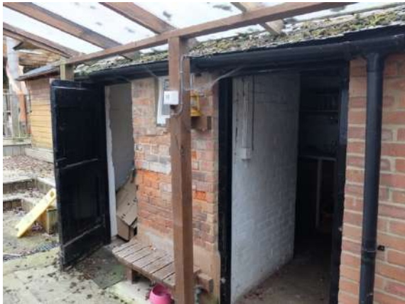
Fig.36- 37 Former stable range used for storage - brickwork showing several phases of construction.
