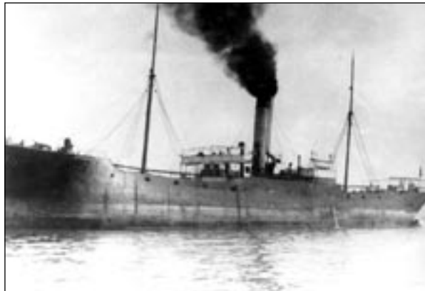
The former SS Deddington, later County of Cardigan
