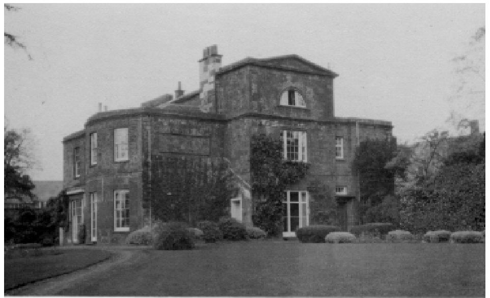
Rear elevation of Deddington Manor from the south west
