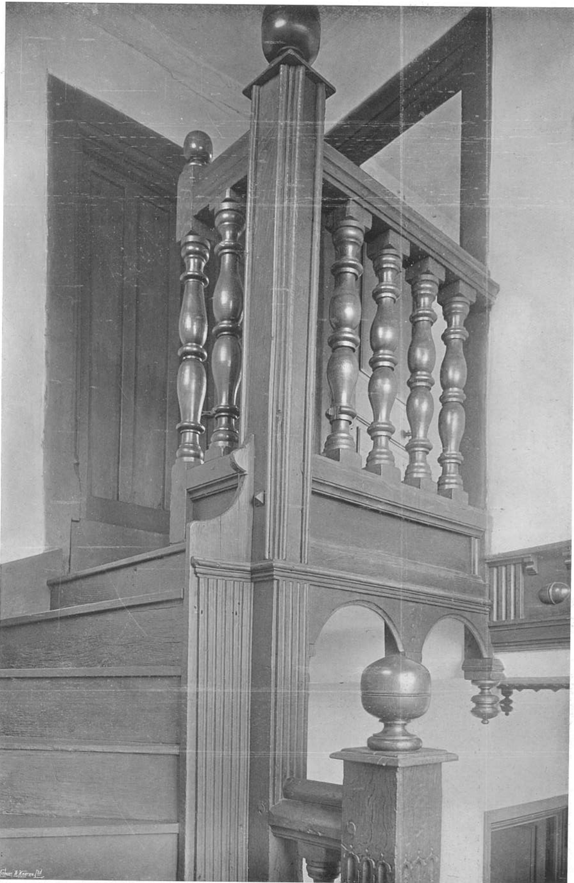
UPPERMOST TREADS OF STAIRCASE, CASTLE HOUSE, DEDDINGTON.
